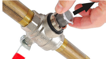
Fig. 7 - taking out the strainer
