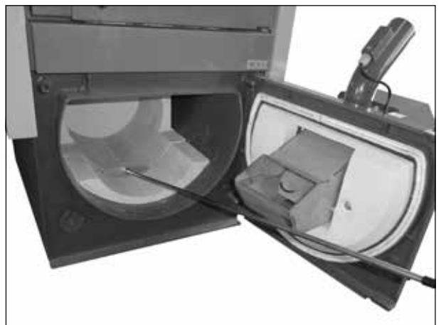
Open bottom door of the boiler during cleaning of the combustion chamber of the boiler when burning pellet.
