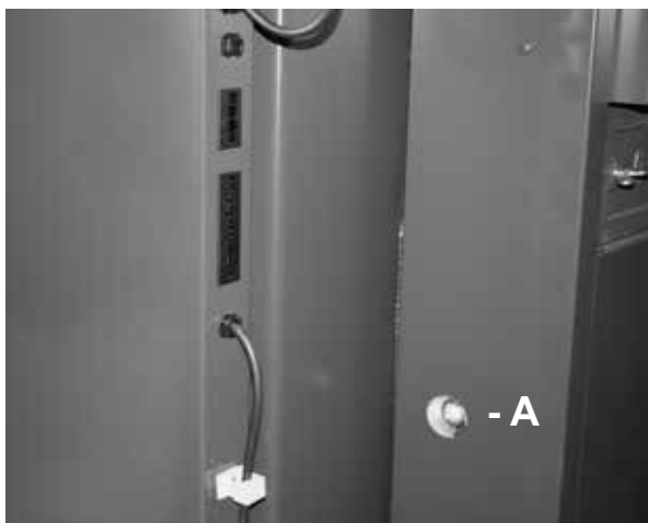
A - hole for to measure actual content (excess) of O 2 when heating with pellets
