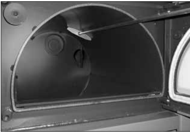
Cleaning the upper stoking chamber with the scraper (poker)
