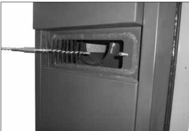
Sample cleaning middle part of the flue way - middle lid
