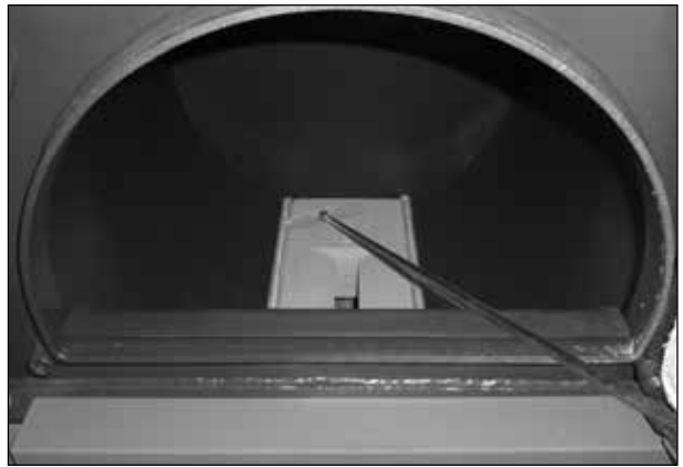
Sweeping the ash through the nozzle down into the bottom (cleaning) chamber. The opening in the nozzle must be always clean and free!
