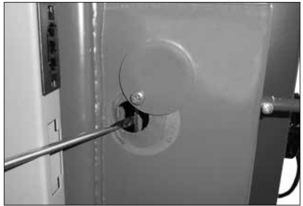
Checking and cleaning regulation of primary-secondary air ratio via cleaning lid
