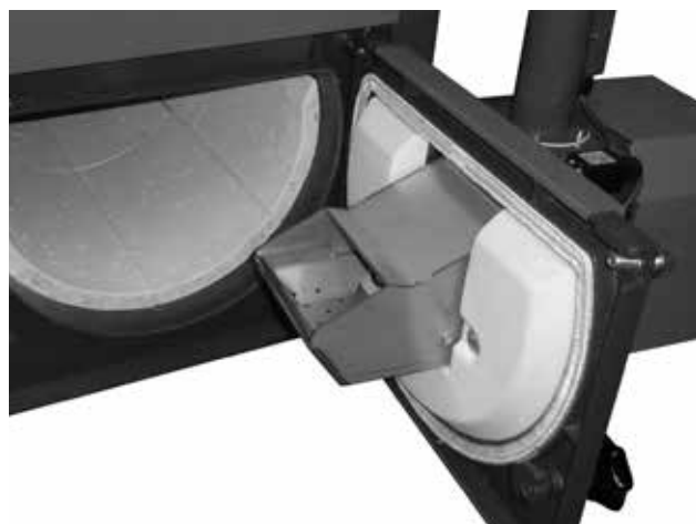
Open combustion chamber of the boiler during cleaning of the combustion chamber of the burner ATMOS A25
