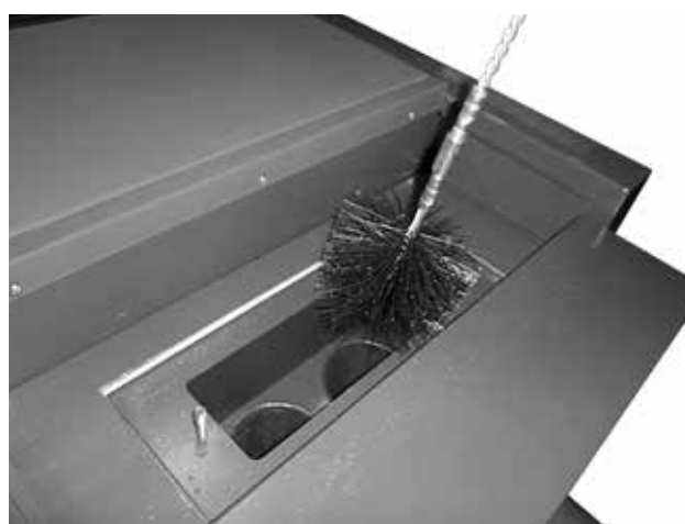
Thorough cleaning of the tube exchanger (tube plates) with the brush
