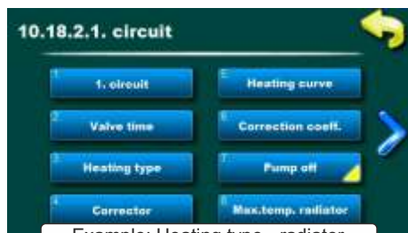
Example: Heating type - radiator
