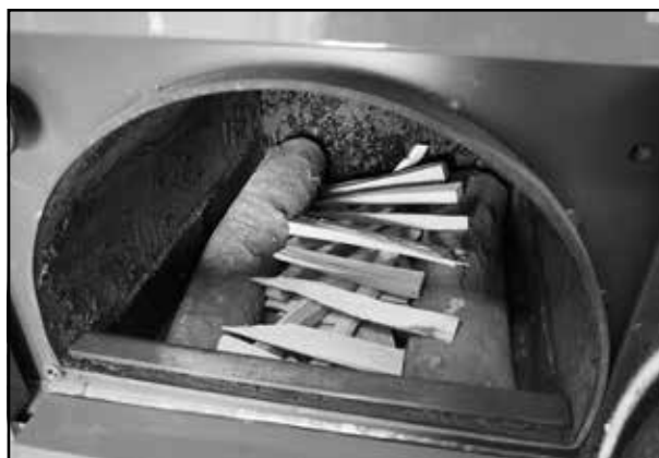
Inserting kindling chips across the chamber above newsprint paper
