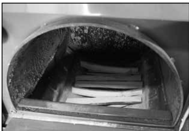
Insertion of the kindling chips perpendicularly to the gasification nozzle opening
