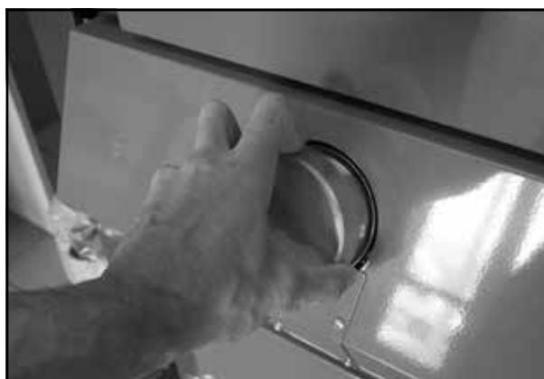
Screwing in and tightening the automatic ignition lid
