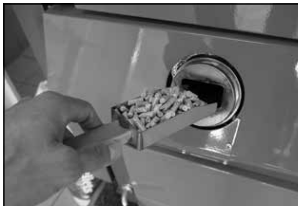
Example of inserting ignition pellets into the ignition chamber
