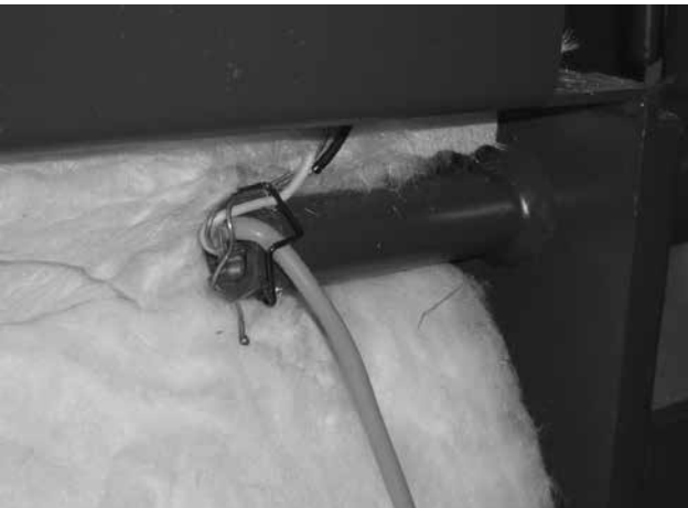
Fig. 15 – View of the water temperature sensor TK in the boiler pocket - boiler with burner in the upper door - DCxxS(X), CxxS, ACxxS, DCxxRS
