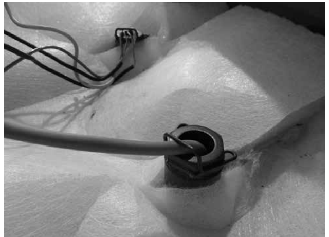
Fig. 16 – View of the water temperature sensor TK in the boiler pocket, DxxP, Pxx type
