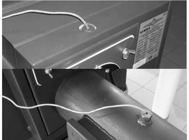
Fig. 14 – View of the flue gas sensor TS or TSV in the flue gas duct pocket. For boilers D30P, D40P and D50P (D45P) is placed on the flue gas channel
