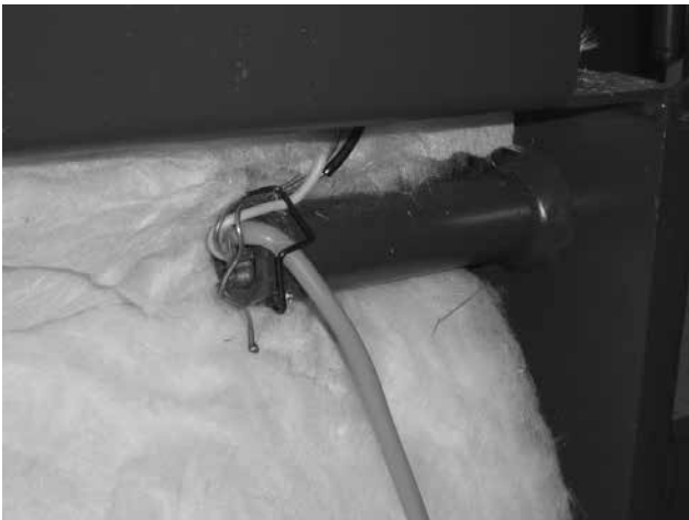
Fig. 15 – View of the water temperature sensor TK in the boiler pocket - DCxxSP(X)/(EP), CxxSP, ACxxSP or boilers with burner in the upper door - DCxxS(X), CxxS(T), ACxxS, KCxxS, DCxxRS
